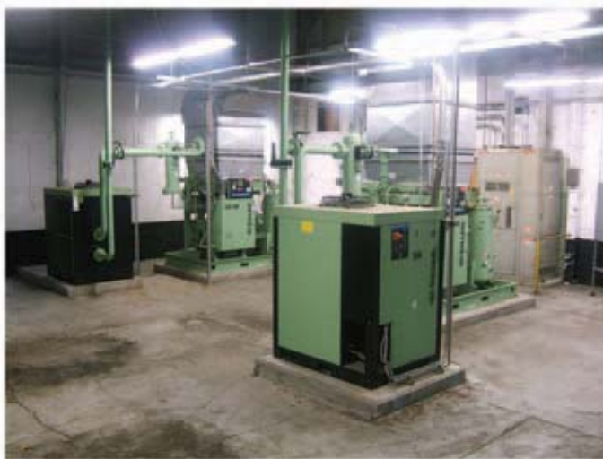
An Industrial Air Centers, Inc. Compressed Air Supply installation that includes compressors, dryers, filters, controlled storage and remote monitoring capability through the internet.
